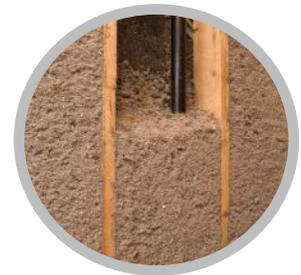
**Cellulose insulation provides seamless coverage**
