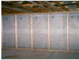
Enviroshield is a dense-pack cellulose insulation system that is intended for application in walls, ceilings and floors behind mesh or poly utilizing Weathershield or ProCell Green insulation.
